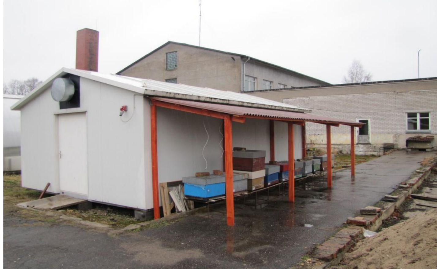
Fig.1. Exterior view of wintering building
